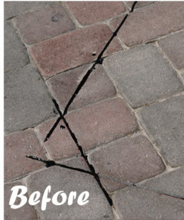
Pavers with Black Sealant
