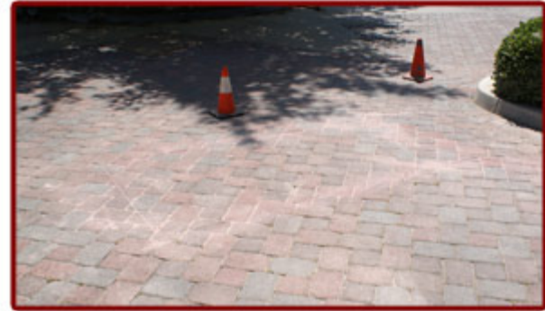
Saw-Cut Tattoo Concealed with Sand
