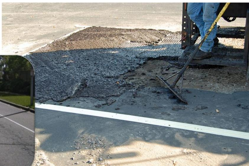
Another issue to consider with putting a loop into a hot asphalt pour is that a water channel will be created around the wire. This can speed up cracks being formed in areas that experience freezing temperatures. Water stuck in the water channel will expand when frozen and contribute to the surface cracking.
